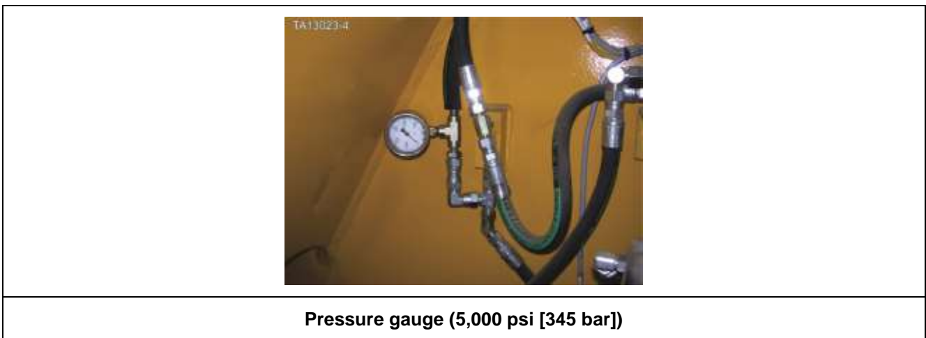
Figure 25. Installed grease supply line pressure gauge
