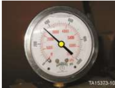
Figure 31. Pressure gauge with correct flow and pressure small flicker at about 350 psi (24 bar)
